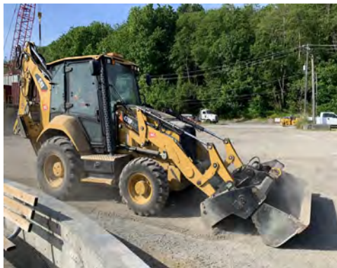
Crews at work
